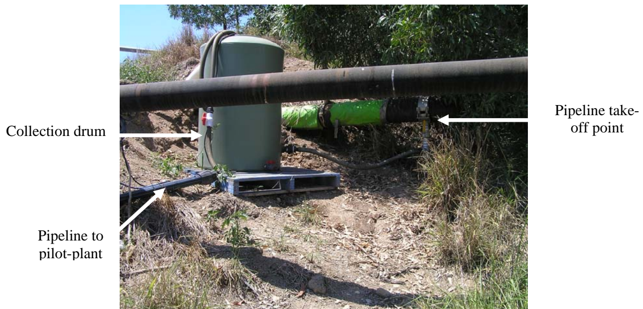
Figure 2.4: Pilot-plant take-off line and collection drum.
