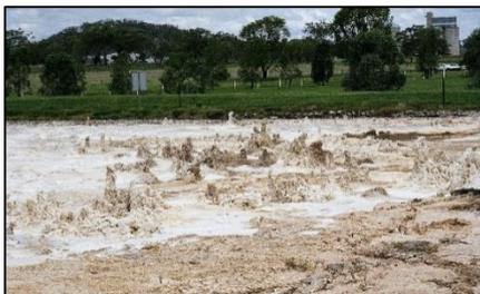
Gas geysers on crusted anaerobic ponds
