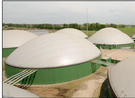
Mixed Vessel Anaerobic Reactor
