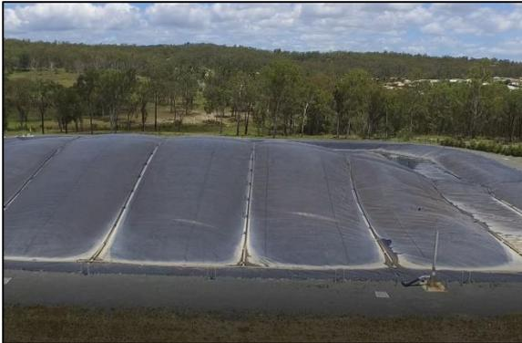
Covered Anaerobic Lagoon or CAL
