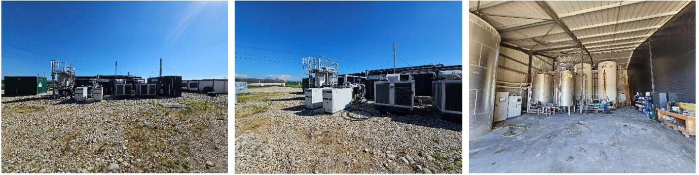
Figure 9. Biomethane Facility at Food Waste Receiving Facility.
