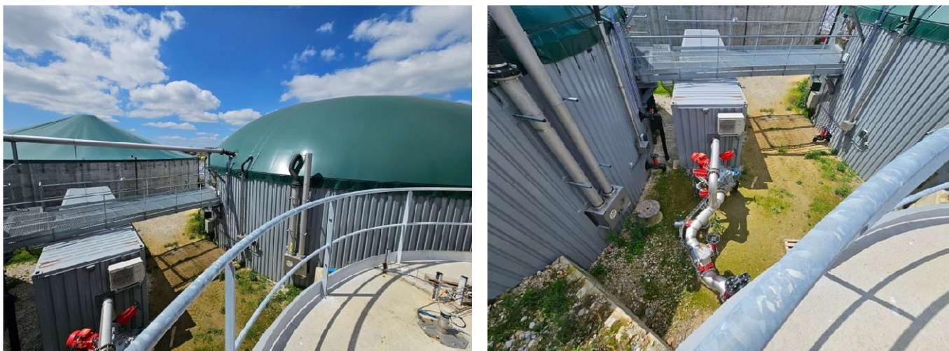
Figure 7. Biodigesters and BioCO<sub>2</sub> recovery from agricultural residues and cow manure as feedstock in France.
