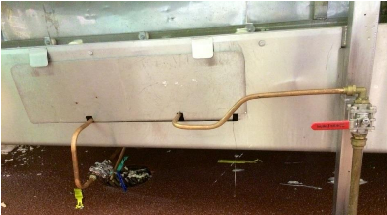
Figure 16. Steam bath tunnel in study two (closed).
