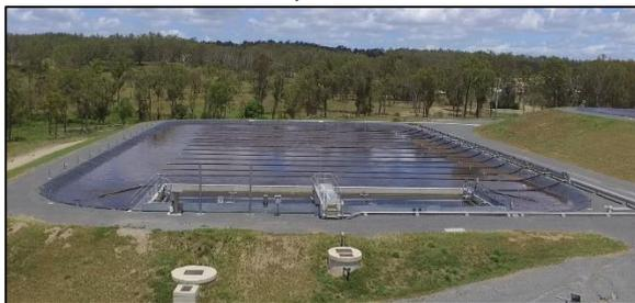
In **Continuous BNR processes**, nitrification and denitrification are performed in different parts of the reactor. An example is the Biolac process where although the denitrification zones are not separated by walls from the nitrification zones, there are distinct areas allocated for each reaction. This requires the constant circulation of flow between zones to complete the reaction.
