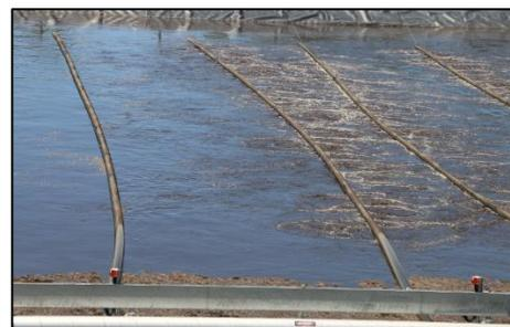
In the Biolac process, the upstream aerated zone provides the nitrate-rich water for the downstream anoxic zone so there is no separate recycle stream. The basin is usually mixed in a manner to minimise the presence of oxygen, for example with submerged mixers.
