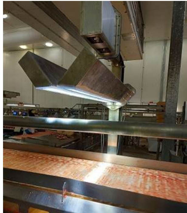
Figure 1: Vision system installed at Oakey Beef Exports
