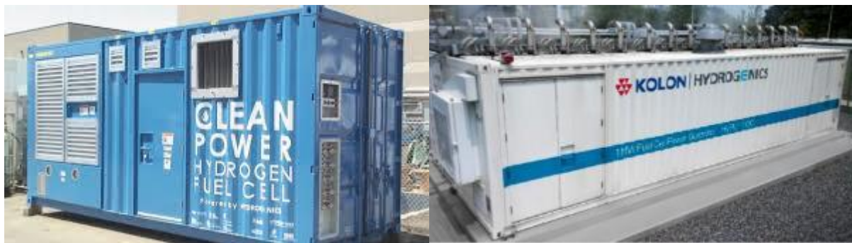
Figure 37: Containerised 200 kW and 1 MW Fuel Cell Modules with Pressurised H 2 Storage 44
