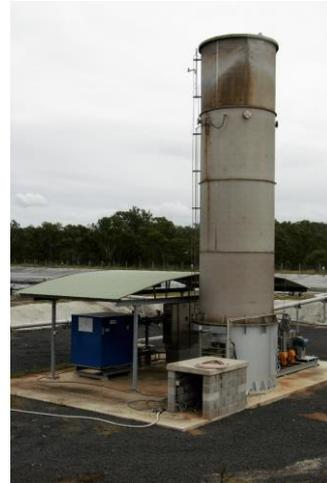
Image 24: Enclosed Biogas Flare
