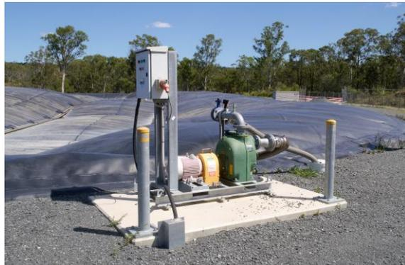
Image 13: Stormwater removal system off CAL cover
