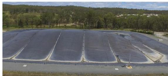
Image 11: Covered anaerobic lagoon
