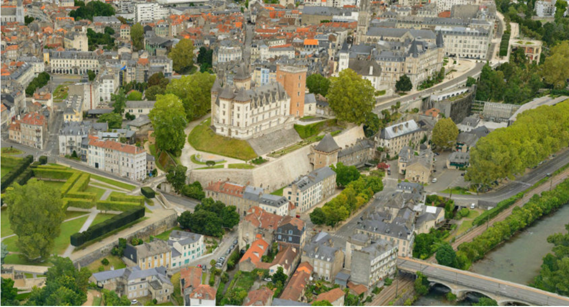
Image 1.1 – hi-fidelity Digital Twin of the French city of Pau, created by Aerometrex from 100,000+ photographs from helicopter, drone, and at street level. Created to preserve the history of the city but also for future construction and infrastructure projects.
